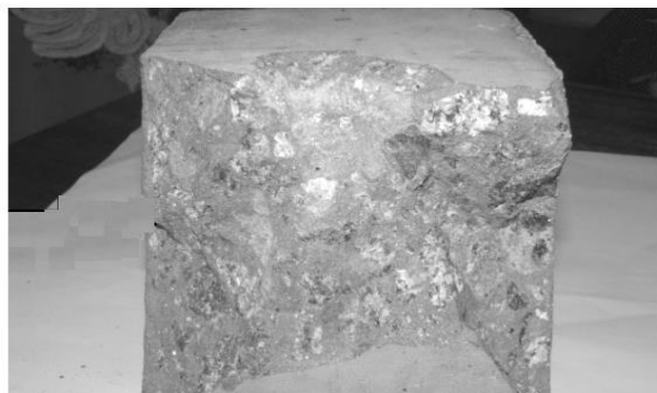
Fig. 6. General composition concrete view (a)
